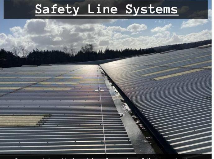
Commercial and Industrial roofs require a fall prevention/arrest system that enables users to work safely, and without restrictions. Our safety line systems are multi-directional and can be fitted to various roofs, regardless of material or size.
